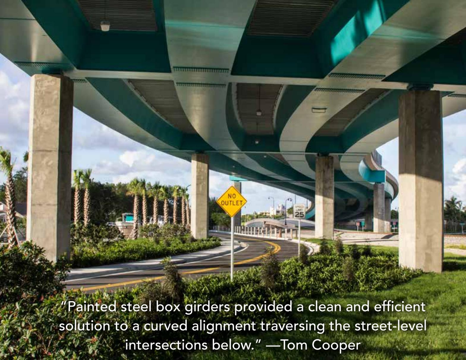
“Painted steel box girders provided a clean and efficient solution to a curved alignment traversing the street-level intersections below.” —Tom Cooper
