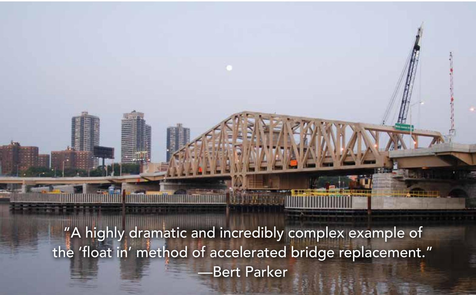
“A highly dramatic and incredibly complex example of the ‘float in’ method of accelerated bridge replacement.”
