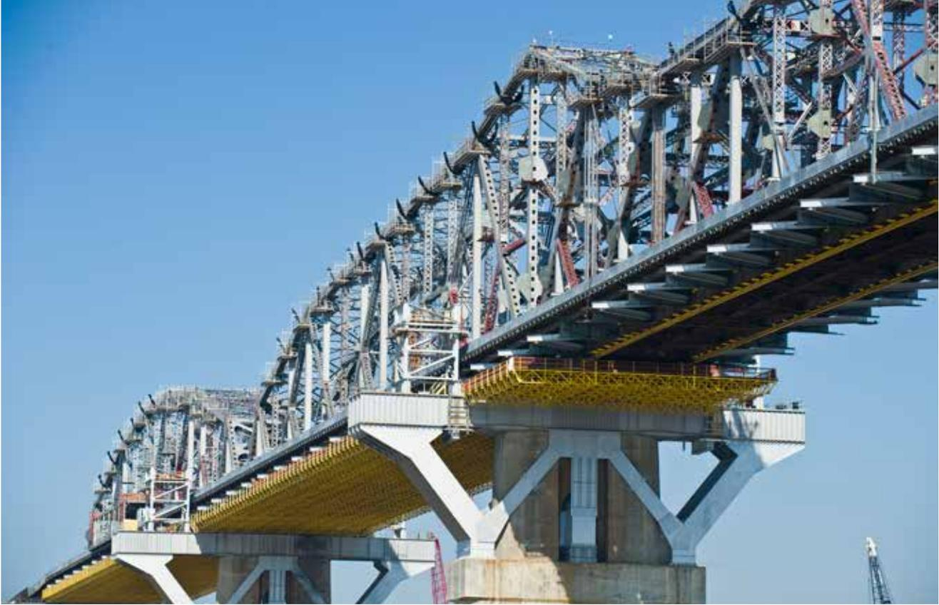
During the first phase, river piers were widened from 60 ft to 80 ft by encasing the lower portion of existing piers with concrete. The encasements supported a new steel “W” frame that was in turn used to support the widening trusses. The 53-ft-tall steel frame is 152 ft wide at the top but only 75 ft wide at its bearings. Once the steel W frame was supported, teams could widen the main river spans.
