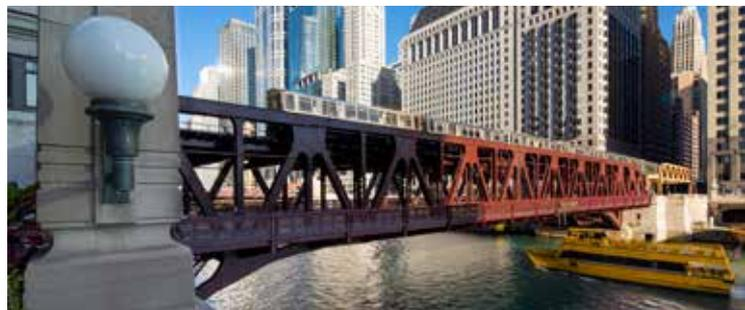
**THE WELLS STREET BRIDGE** is the longest double-deck, double-leaf, bascule bridge built over the Chicago River, and only one of two remaining bascule bridges in the city of Chicago that carries both automobile and transit (Chicago Transit Authority elevated trains) on two levels.
