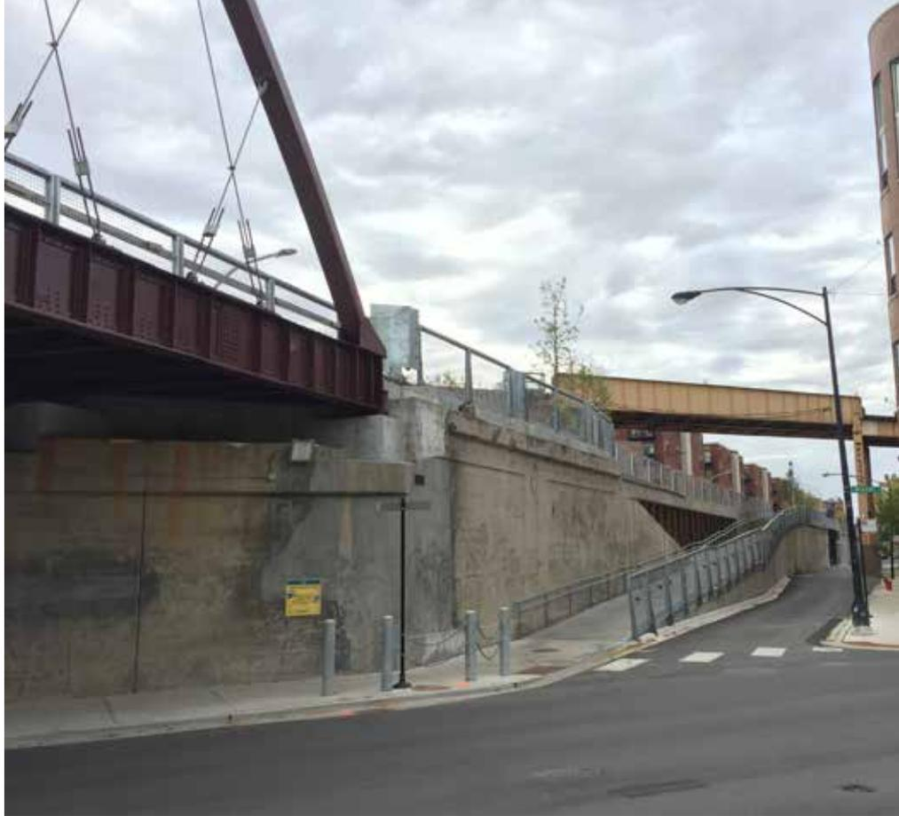
the trail at Milwaukee Avenue and moving inward and upward until access to the trail was gained. Tied-back steel sheet pile wall was incorporated to accomplish this feat.
