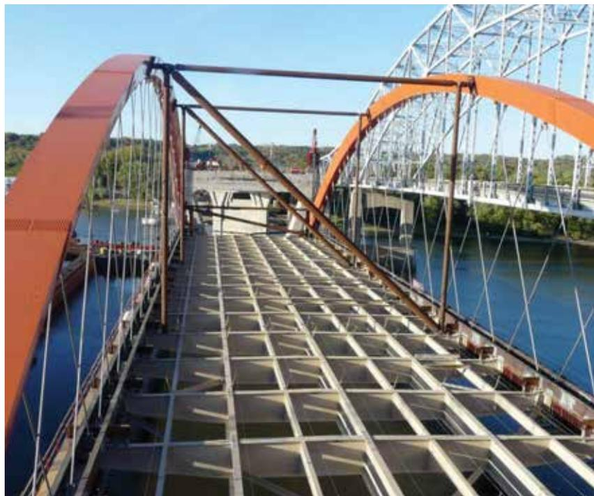
The SPMTs under the corners at each end were connected together to act in unison for moving the arch system transversely down to the river bank and over a trestle onto barges. Water level monitors at each corner of the arch were used to check the slope between the ends of each arch and the SPMTs were adjusted vertically to maintain a constant slope between the arches and avoid twisting the floor system as they marched the arch down a 3.5% slope to the river and onto the barges.
