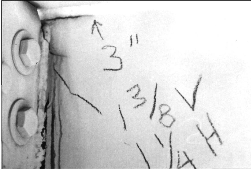
Fig. 35 Fatigue Cracks at Floor Beam Connection Plate Web Gap
