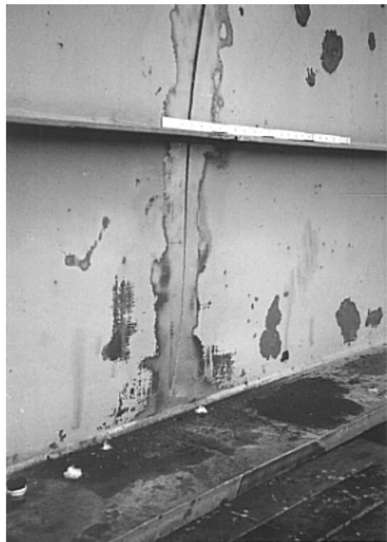
Figure 44 Crack in Girder Web from Splice in Longitudinal Stiffener
