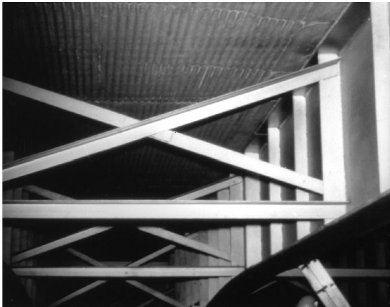
Fig. 33 X-Bracing and Girders
