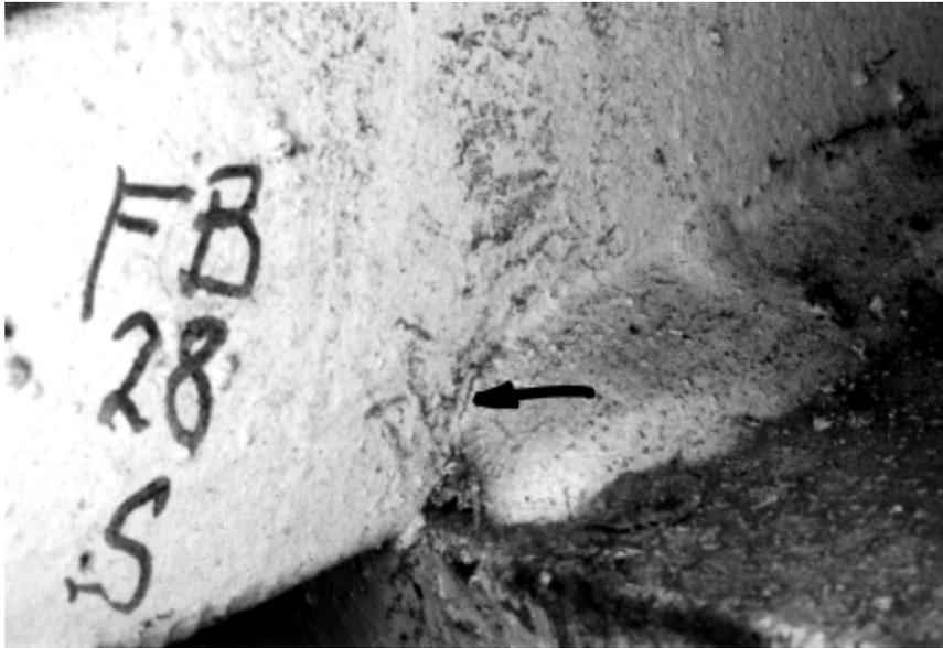
Figure 43 Fatigue Crack at Lateral Gusset Plate Welded to Floor Beam Web
