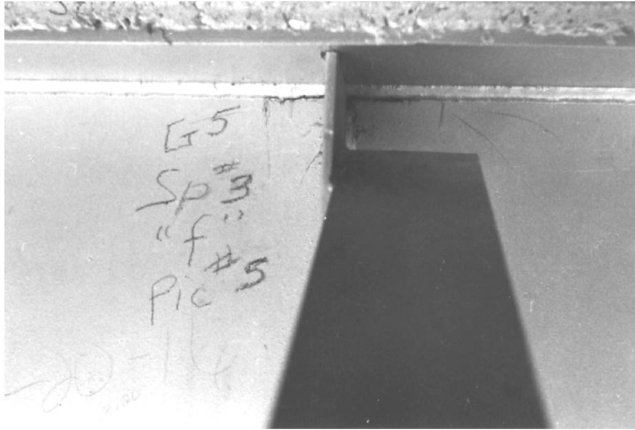
Fig. 34 Fatigue Cracks in Web Gap of Diaphragm Connection Plate
