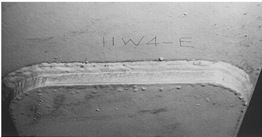
Figure 41 Fatigue Crack at End of Cover Plate
