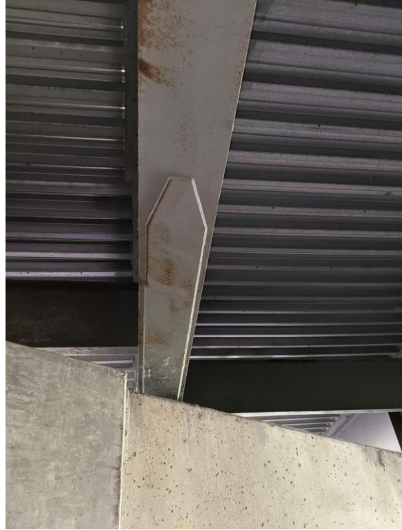
(b) edges of cover plates and undersides of bottom flanges
