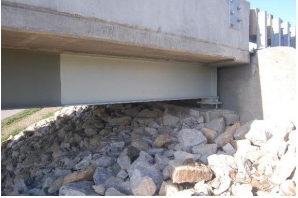
(a) girder end at an abutment
