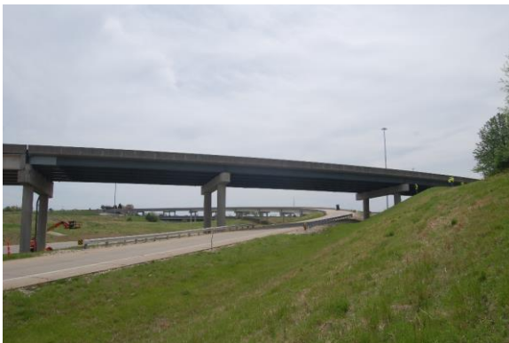
(c) large vertical clearance over a roadway
