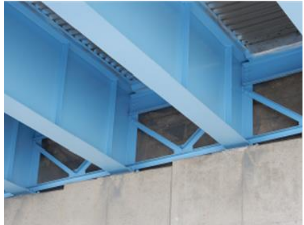
Figure B27. Photo. Example of view of bearing location.
