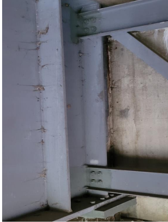
(b) properly field coated bolted connection
