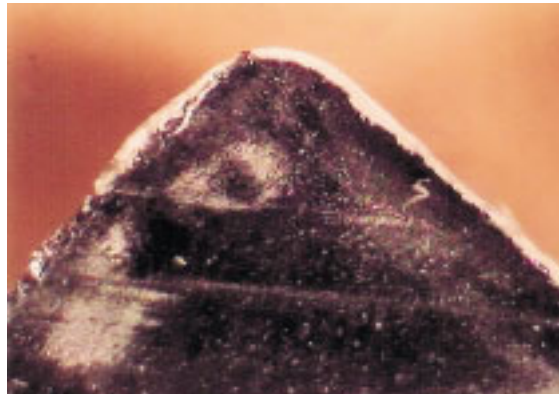
Phase 1, Photograph 26 Industrial Enamel (single coat) Corner MR-0 (90°)
