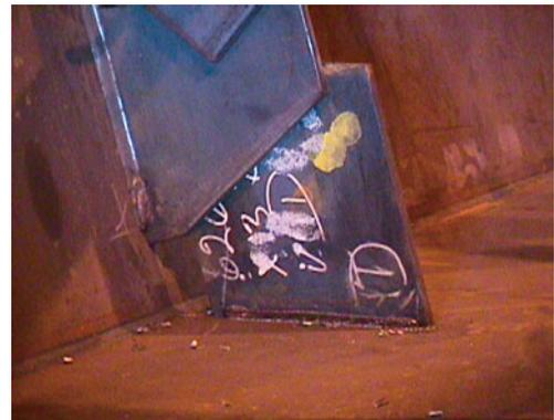
Figure 11: Stiffeners to which bracing members are attached should be connected to girder flanges to reduce local distortion. Shown is a typical detail for connection to the bottom flange.
