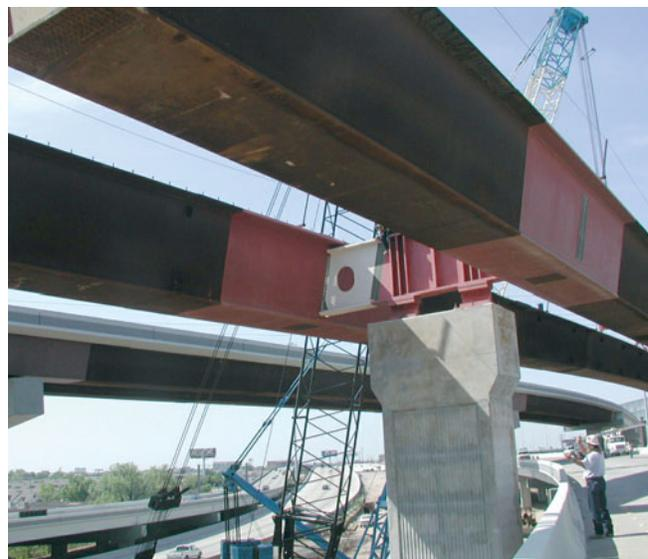
The effects of transverse loading on the weld because of web slope and lateral bracing loads should be included...
