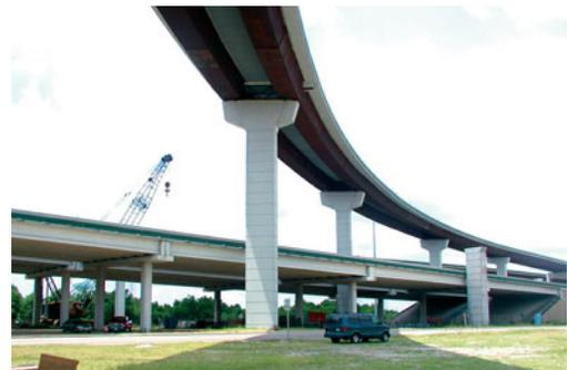
Figure 5: Simple lines, smooth surfaces, and fewer parts visible; the clean appearance of tub girders offers distinct aesthetic advantages.
