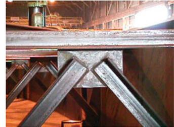
than 1-inch thick to determine whether practical stiffness needs are met. In no case should bottom tension flanges be less than 1/2-inch thick. Another suggested guideline is that the bottom tension flanges have a b/t ratio of 80 or less.”
