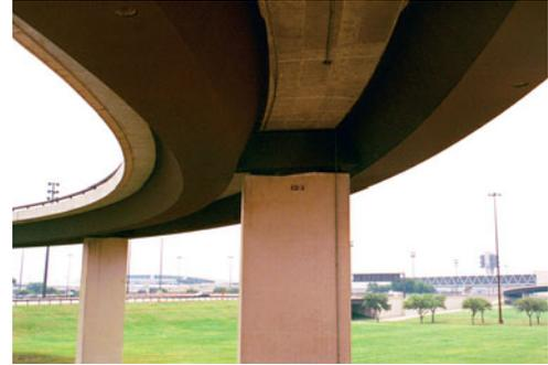
Figure 4: Steel tub girders built on horizontal radii as tight as 175 feet were constructed at the Dallas/Fort Worth International Airport in the late 1970s.
