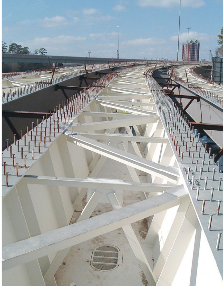
Internal intermediate diaphragms are provided in tub girders to control cross-sectional distortion, which introduces additional stresses in box girders and should be minimized...
