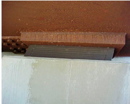
*Figure 23: The simplicity of steel-reinforced neoprene bearings illustrated in an expansion bearing at the end of an 880-foot continuous tub girder unit*
