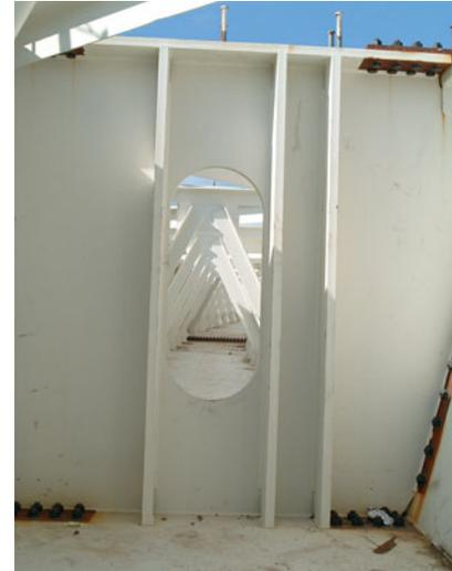
Figure 13: Internal diaphragms at supports generally use full-depth solid webs, with access manholes between the bearing stiffeners.
