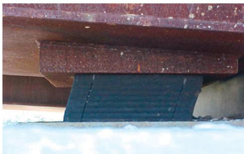
Figure 17: Steel-reinforced neoprene bearings are a simple, low-maintenance bearing option.
