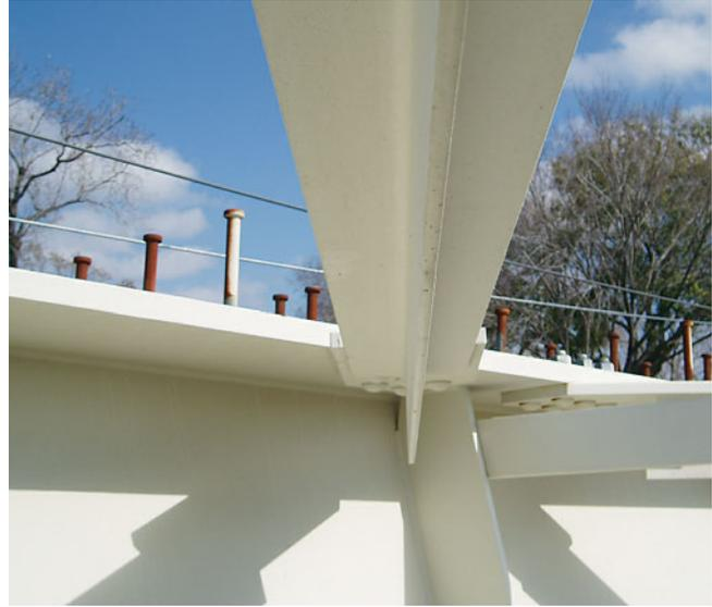
Top flange lateral bracing is required in tub girders to form the “fourth side” of the box until the slab is in place...
