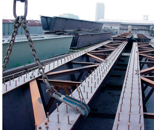
Overall width of a bridge is also a controlling factor in setting individual tub girder widths and spacings...
