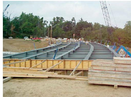
Figure 3: For slight curvature and spans below approximately 120 feet, other superstructure types, such as the curved steel plate girders in this shallow depth curved grade separation bridge, may be a better choice than steel tub girders.
