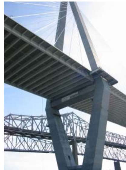
Successful large steel design/build project: Cooper River bridge in Charleston, SC—completed within budget one full year ahead of schedule.
