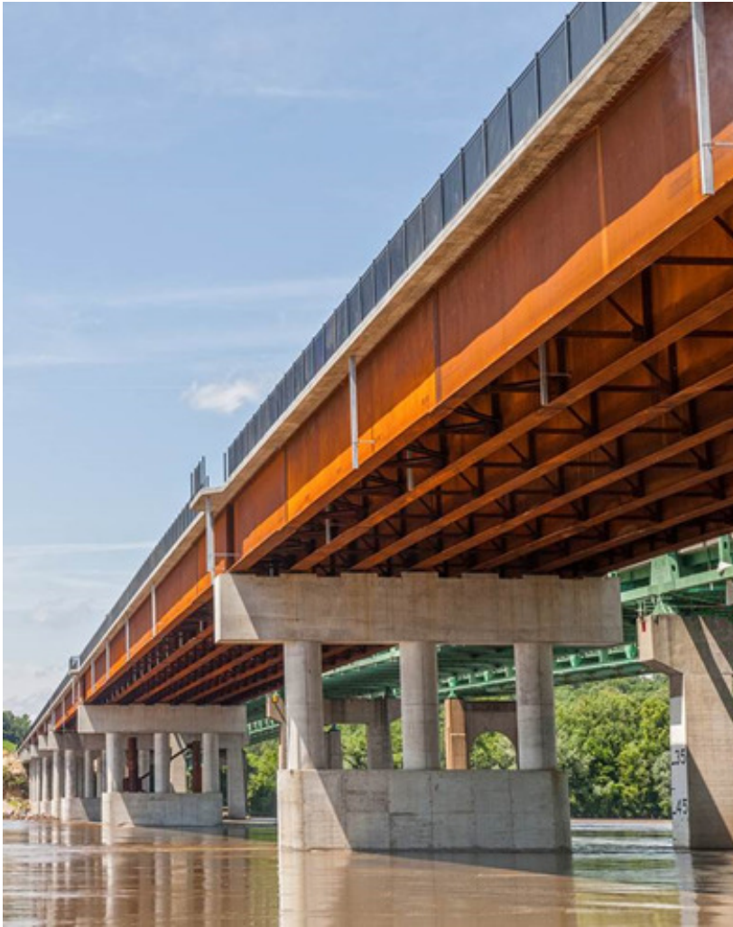
Photo courtesy of Burns & McDonnell
