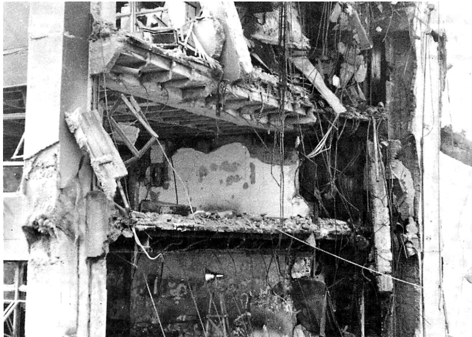
Figure 7. CESP 2 Core Collapse in Sao Paulo, Brazil
