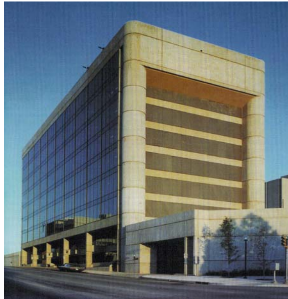
Figure 2. Alfred P. Murrah Federal Building in Oklahoma City Before Explosion
