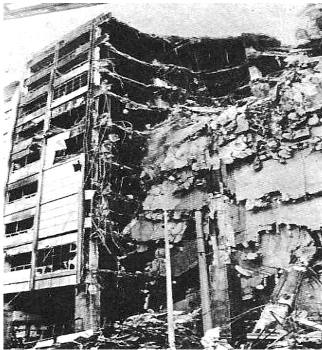
Figure 9. Katrantzos Building in Athens, Greece After 1980 Fire
