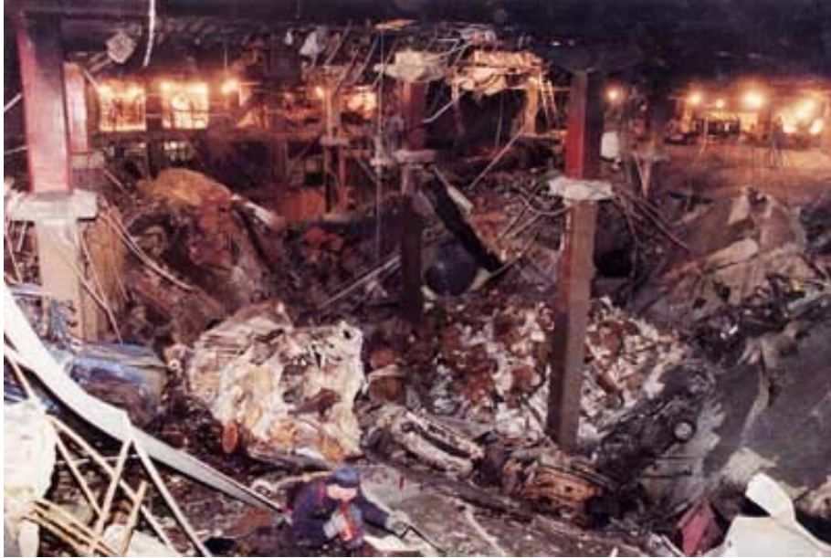
Figure 1. Destruction of Floor Slab Bracing and Weakened Lower Columns in WTC 1 after February 1993 Explosion (from Bureau of ATF 1993 explosives incident report)
