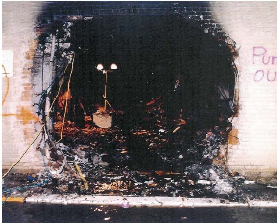
Figure 12. Impact Exit Hole at AE Drive Wall in Pentagon
