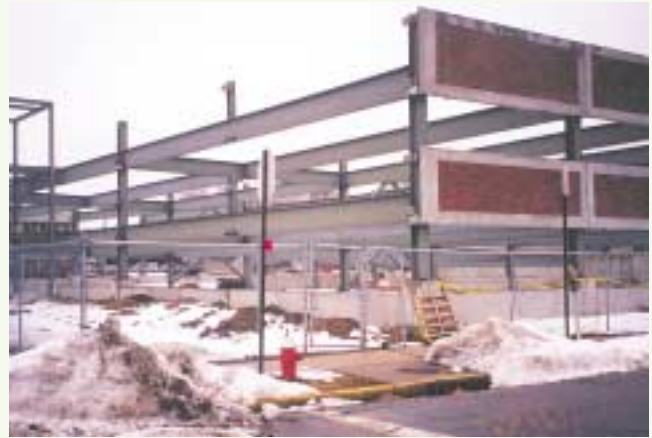
Winthrop University Hospital, Mineola, New York 630 spaces - Carl Walker Construction Group Post-tensioned deck on steel frame
