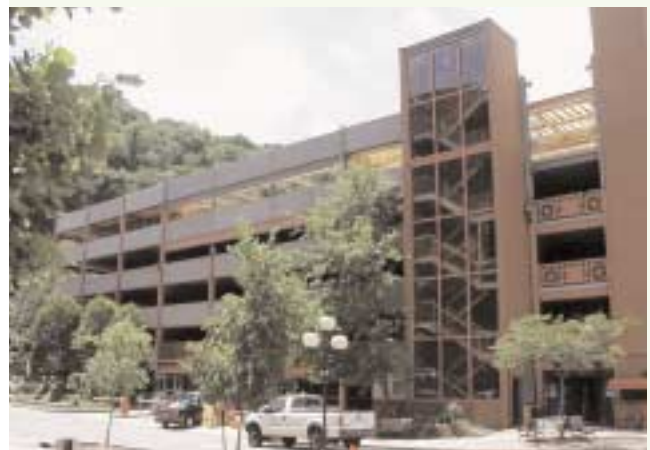
Station Square Pittsburgh, Pennsylvania Original structure: 800 spaces Expansion added: 400 spaces
