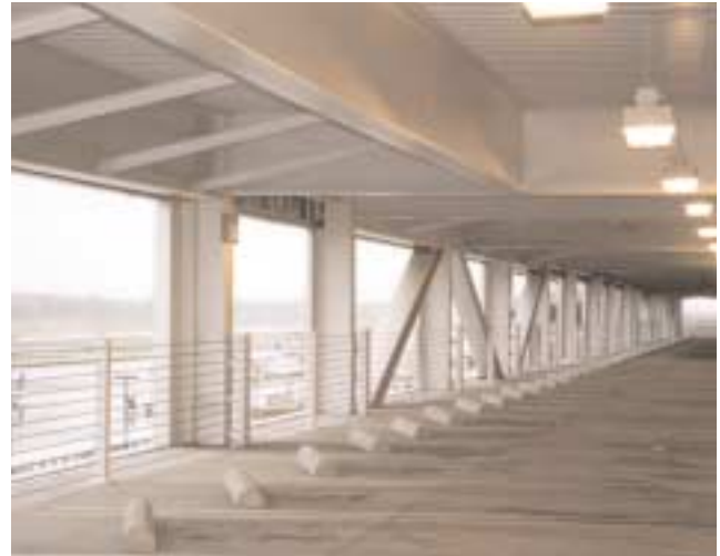
Portland International Airport 3,300 spaces added KPFF Consulting Engineers & Zimmer Gunsul Frasca Architects
