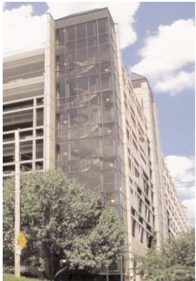
Allegheny General Hospital Pittsburgh, Pennsylvania 1,100 spaces Mulach Parking Structures
