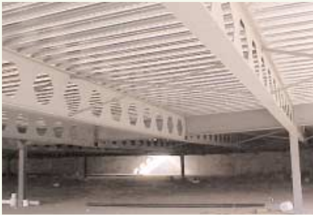
Crickelwood Hill Apartments - Built in 1974 Pittsburgh, Pennsylvania Mulach Parking Structures Post-tensioned deck on steel frame
