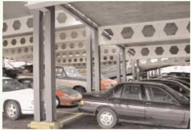
Crickelwood Hill Apartments - Built in 1974 Pittsburgh, Pennsylvania Mulach Parking Structures Post-tensioned deck on steel frame
