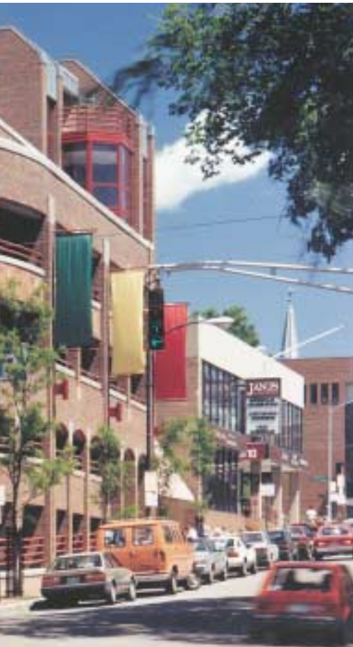
Harvard Square Parking Garage Cambridge, Massachusetts 215 spaces Maguire Group
