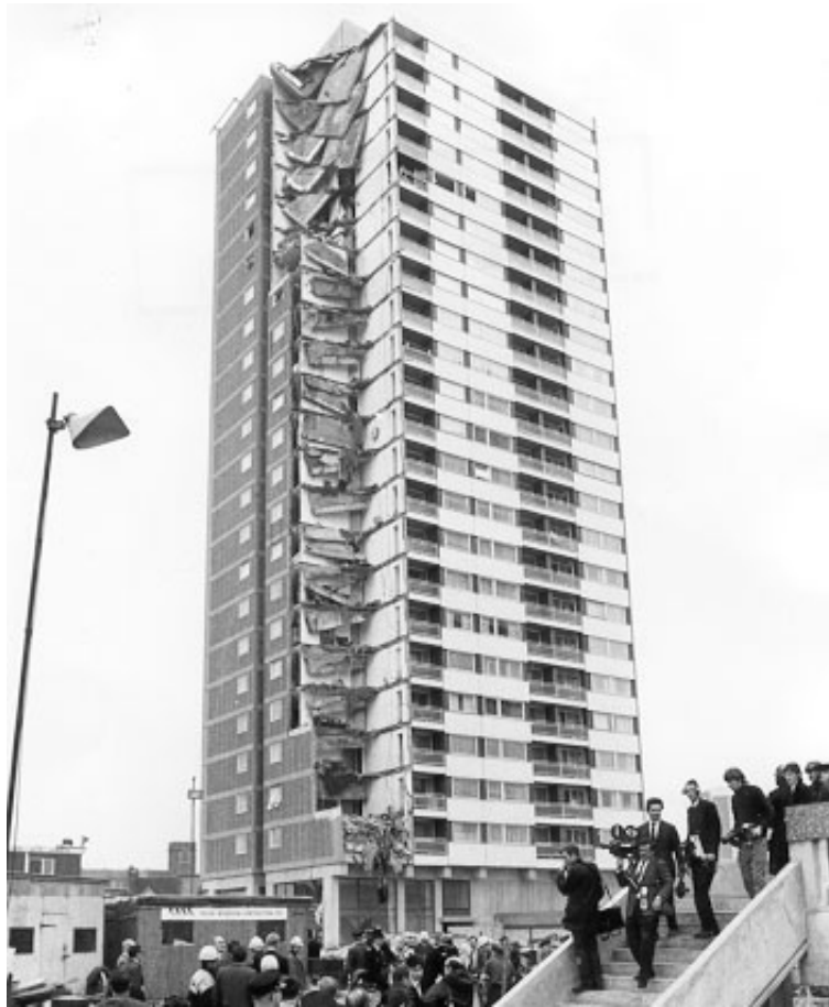
Fig. 1. Ronan Point building after 16 May 1968 collapse
