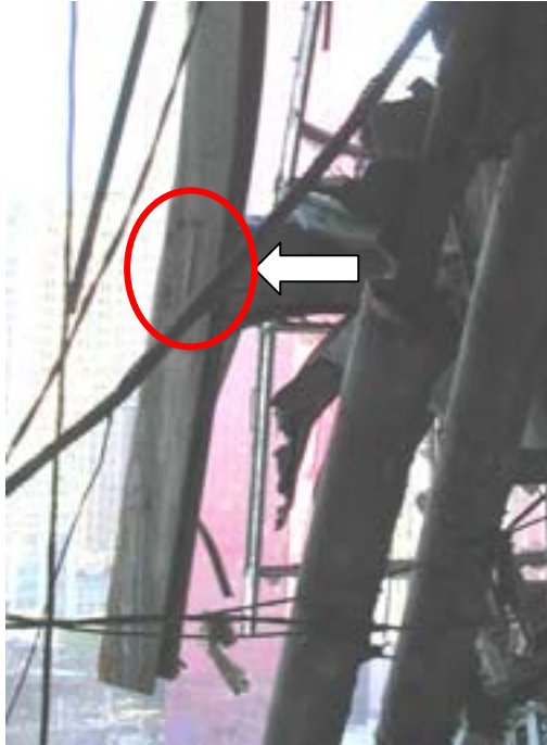
Figure 15 - Failed beam-column connection in Deutsche Bank Building
