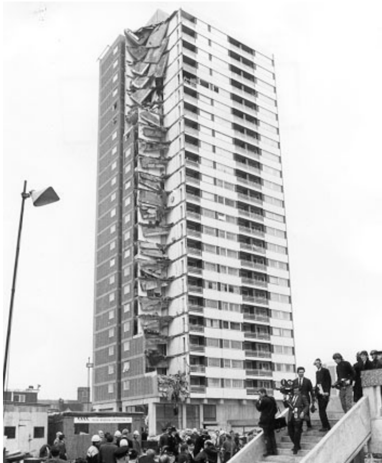
Fig. 1. Ronan Point building after 16 May 1968 collapse
