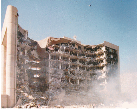
a. Murrah Federal Building
