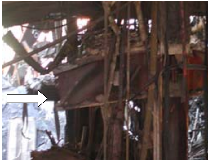
Figure 16 - Failed bolted high strength shear connection in World Trade Center 5
