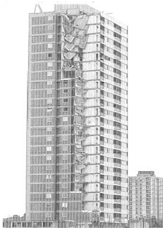
Figure 1 Post-Incident View of the Ronan Point Building (HMSO, 1968)
