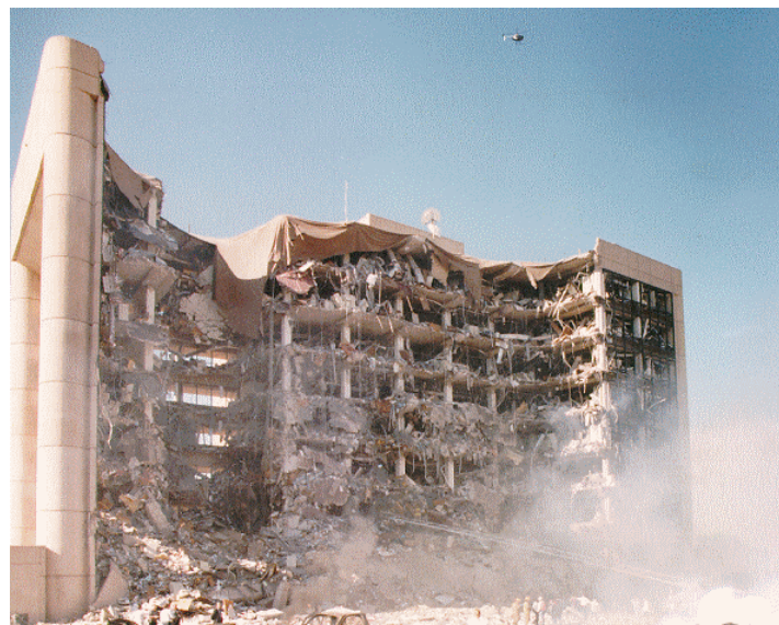
Figure 2 - Remains of the Murrah Building after blast-induced progressive collapse
