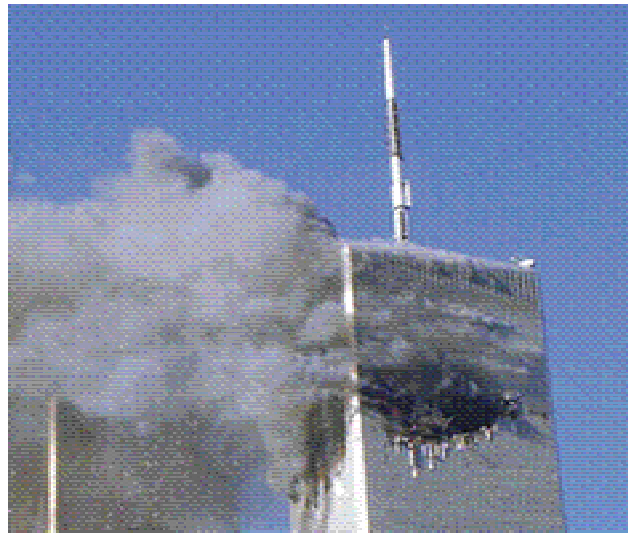
Figure - 3. North Tower of World Trade Center, Illustrating the ability of the perimeter frame to bridge around the massive aircraft impact damage and arrest progressive collapse.
