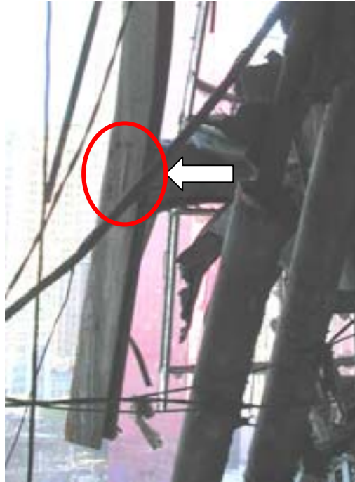
Figure 15 - Failed beam-column connection in Deutsche Bank Building
