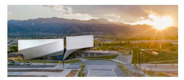
**Distinct aesthetic:** The façade's 9,000 panels evoke an athlete's wardrobe. Each panel has unique connections of exterior walls to roof and floor elements – all accommodated more easily with a custom clip.
