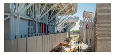
**Solar shading:** The steel-framed solar structures, with patterns inspired by the shape of human DNA, shade the central "Agora" while generating 20% of the campus's energy needs, merging functionality with educational design. The Agora is designed to maintain a peak temperature of 85 degrees in the desert heat.
